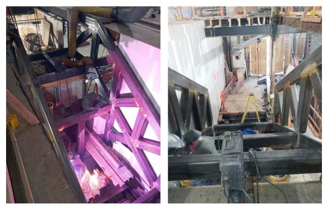
Principal Dean Speranza of Nouveau Elevator was tasked by Target to solve a major problem at 606 West 181st Street. The issue was installing two escalators in the existing space with minimal clearances available throughout. The company looked at every possible location for the installation of these units, keeping in mind that there was limited space below the top floor for structural support of the top pits.
